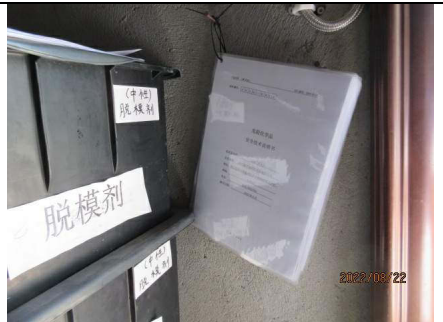
Photo 38) MSDS posted at chemical storage area
